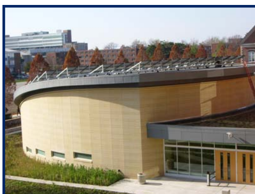
Pictured here, the solar panels and drought-free rain garden on the Business Instructional Facility’s roof are two of the new green building’s many sustainable features. The new facility uses 50% less energy than a comparably sized building.
